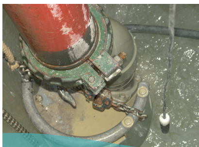
Building site pumps
